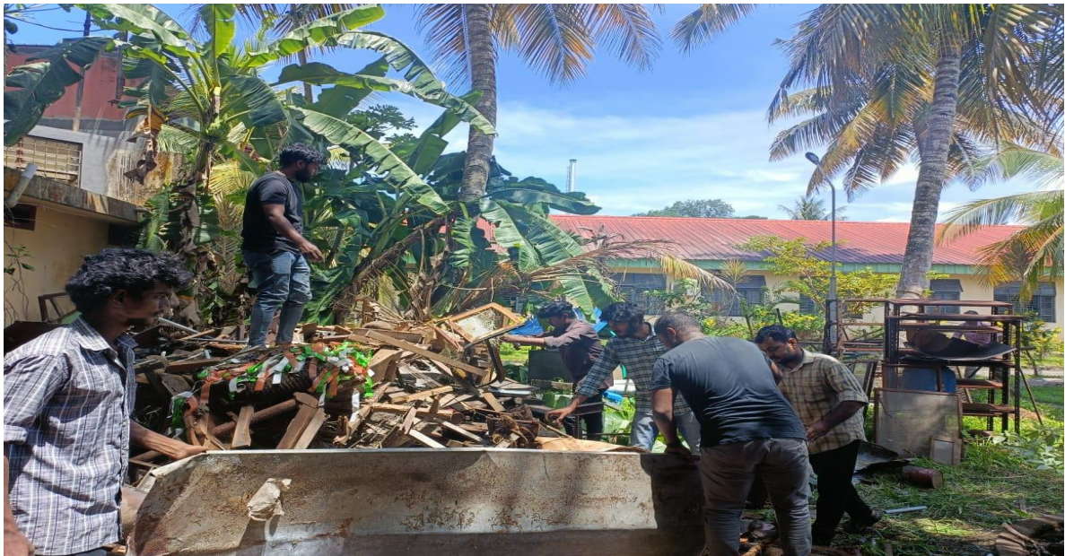
Cleaning In Progress
