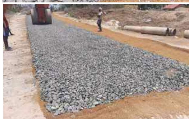
NIT Trichi - Laying and rolling of aggregate
