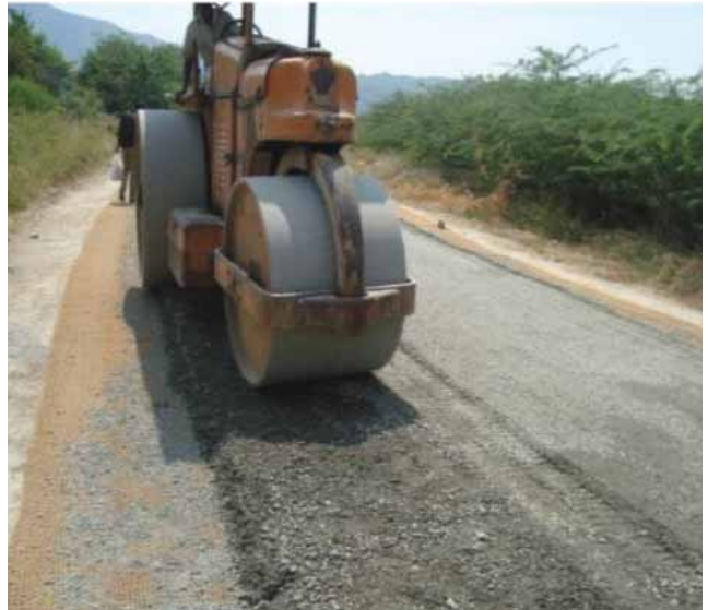
COMPACTING GSB LAYER WITH ROAD ROLLER
