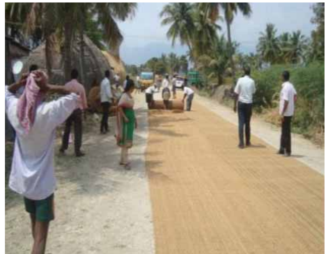
LAYING OF COIR GEOTEXTILE
