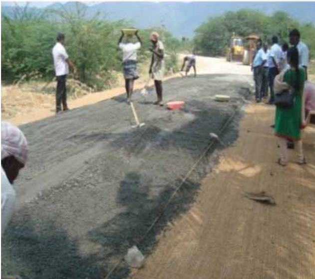
LAYING OF GSB OVER COIR GEOTEXTILE
