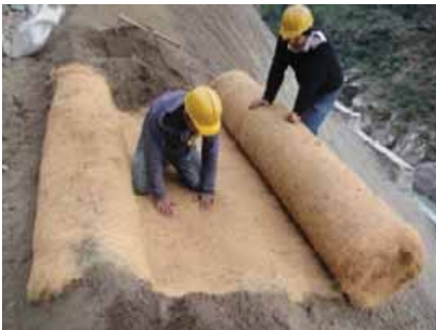
Figure 8: Laying and anchoring of BioMac® CC
