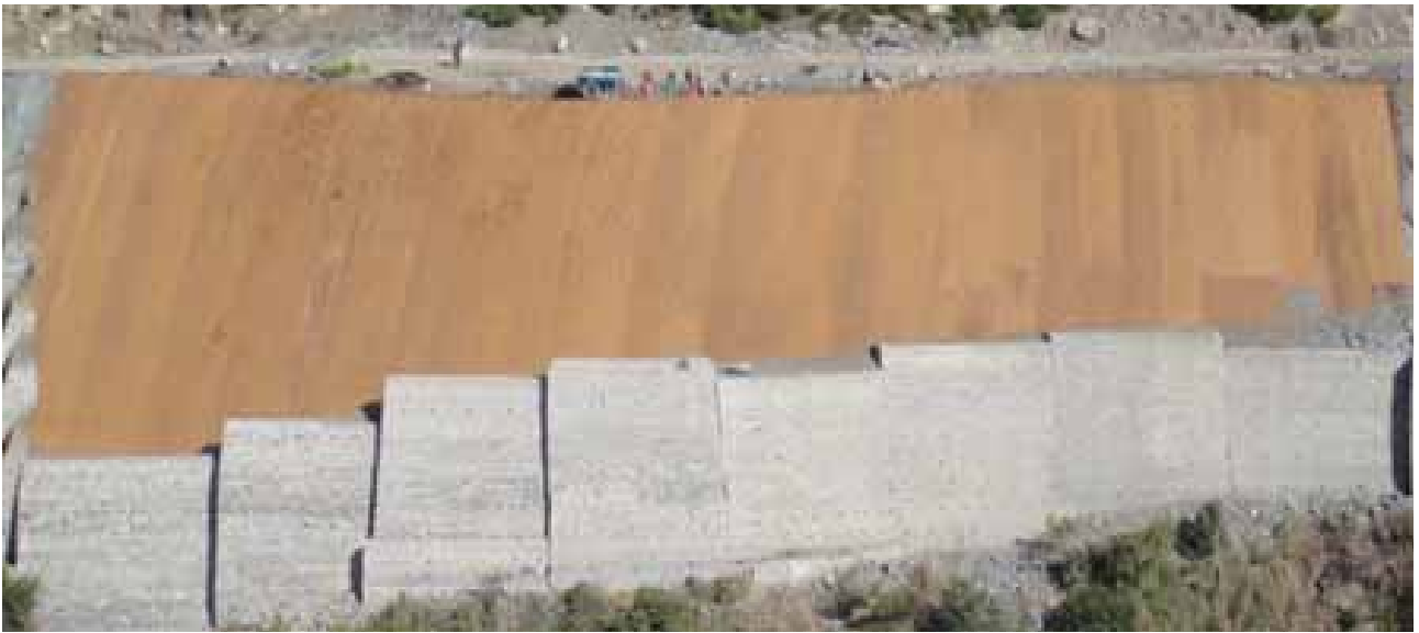
Figure 9: Site condition after installation of 'BioMac® CC'
