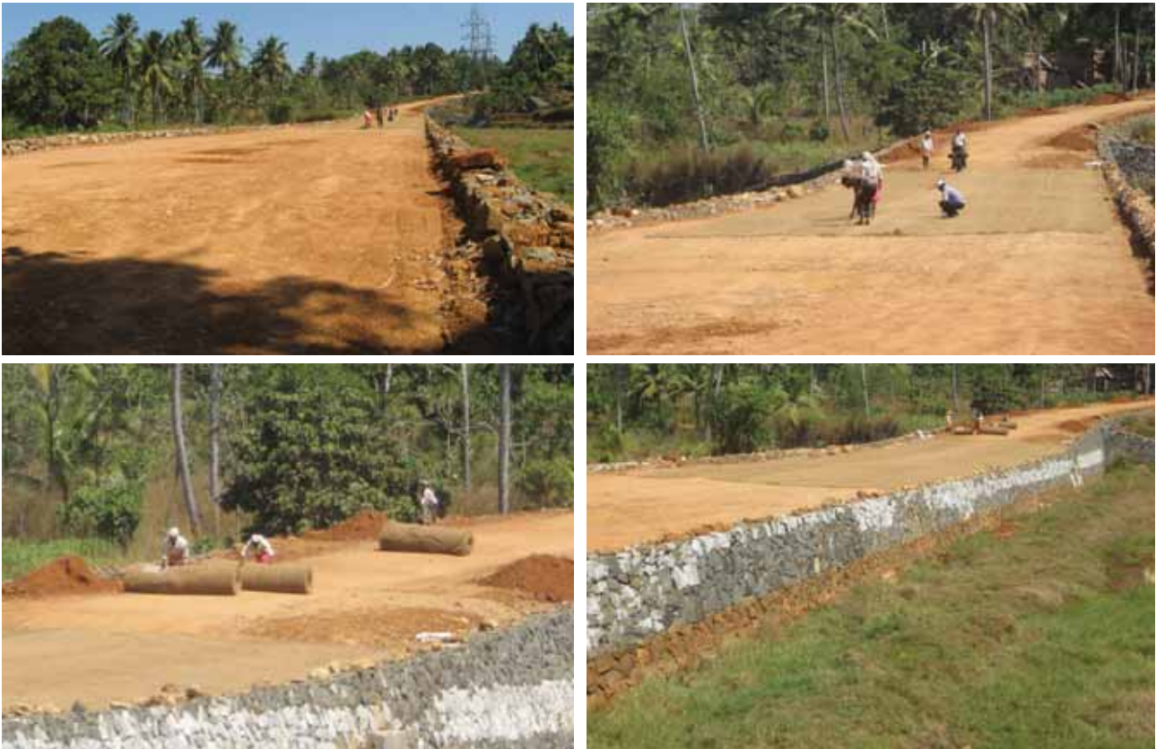
Fig:2 Construction of Coir geotextile Reinforced Pavement
