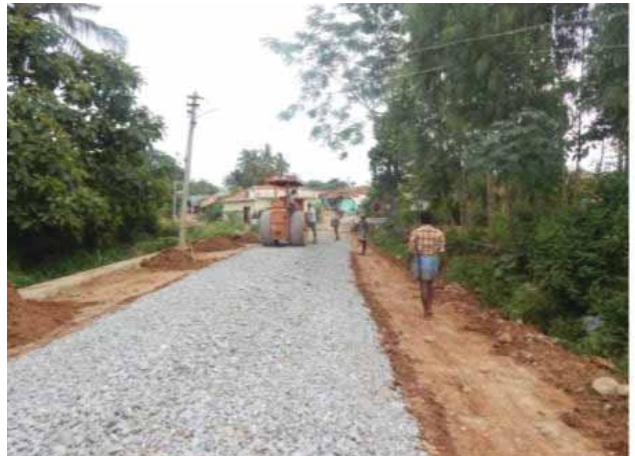
COMPACTING WBM LAYER WITH ROAD ROLLER
