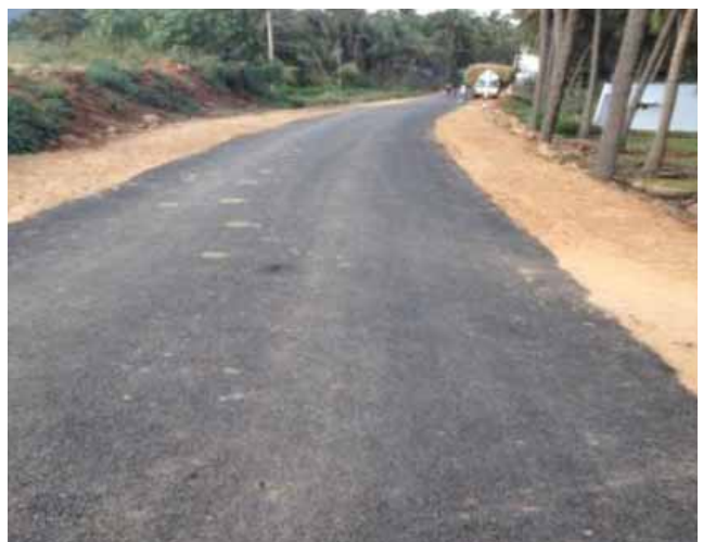
FINISHED COIR GEOTEXTILE REINFORCED PAVEMENT
