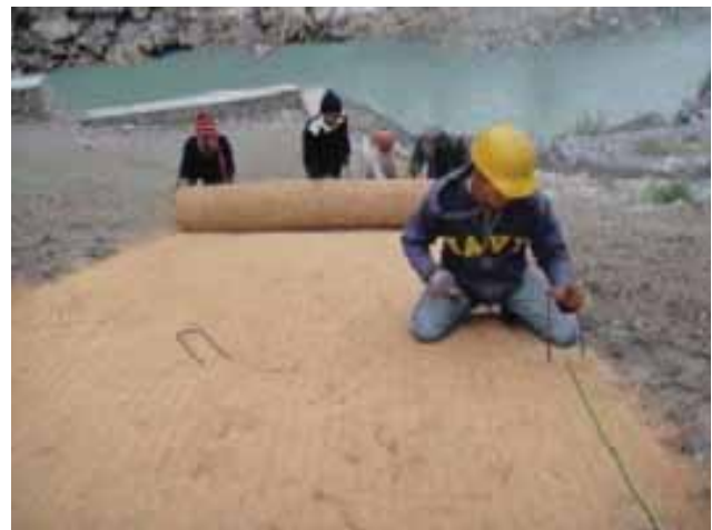
Figure 8: Laying and anchoring of BioMac® CC
