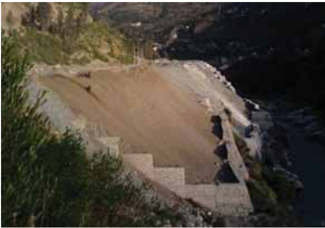
Figure 10: (a) Site condition during installation of 'BioMac® CC' (b) vegetated slope
