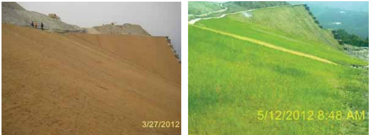
Figure 13: Slope protected with ‘Biomac CC’ (a) after installation (b) 9 months after installation
