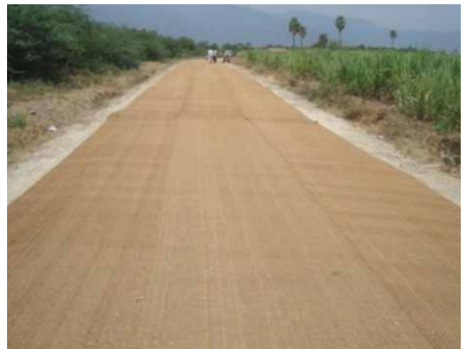
COIR GEOTEXTILE READY FOR SUB-BASE
