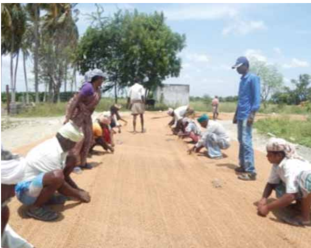
TYING OF COIR GEOTEXTILE ROLLS
