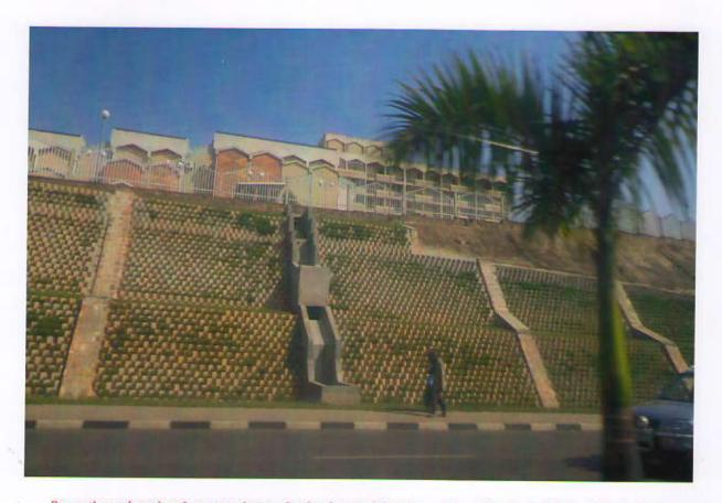
Presently used product & green technique for the slope stabilization cum beautification in Kigali – Rwanda & the Parliament Building is atop; the cost effective coir geo-textile can effectively substitute the present system
