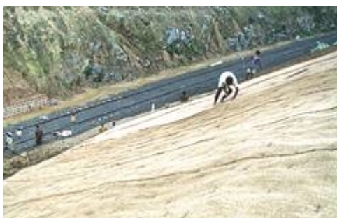
Protection of Rail Embankment (Konkan)
