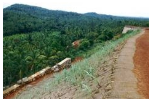
Protection of Road Embankment (IIM(K) – Kozhilode)
