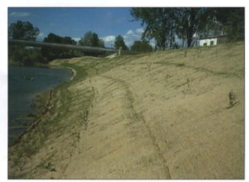
The coir logs used on the project are composed of shredded coconut husk fiber packed at 144 Kilograms per cubic meter (9 pound per cubic foot) into polyethylene mesh netting exterior. They are 30.5 centimeter (12 inch) diameter cylinders, 6.1 meters (20 feet) in length and weighing 65.3 kilograms (144 pound) each when dry.
