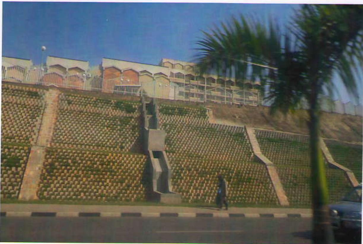
Presently used product & green technique for the slope stabilization cum beautification in Kigali - Rwanda & the Parliament Building is atop; the cost effective coir geo-textile can effectively substitute the present system
