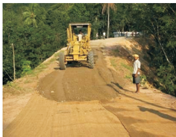
Spreading of soil
