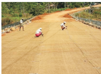
Fixing of laid coir geo textiles
