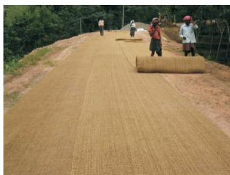
Laying of coir geo textiles
