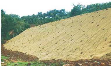
Coir geo textiles laid road embankment
